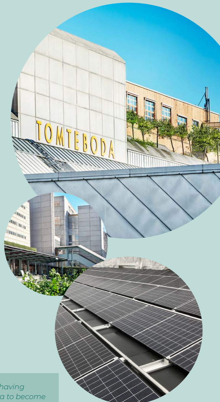
Large-scale solar panel installation at the roof of our Tomtebodan asset in Solna, Stockholm.
